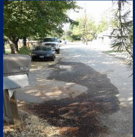
Overflow from clean out
