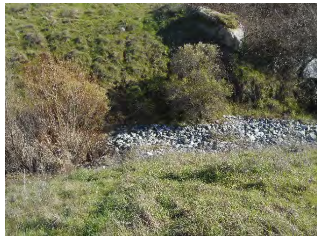
Figure 13 Red Ravine erosion control rip rap on south reach
