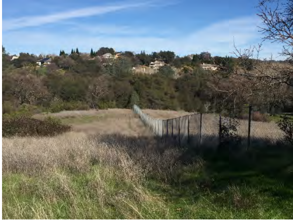
Figure 6 Existing Chain-Link Fence on Perimeter
