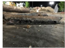
FOG Related Corrosion
