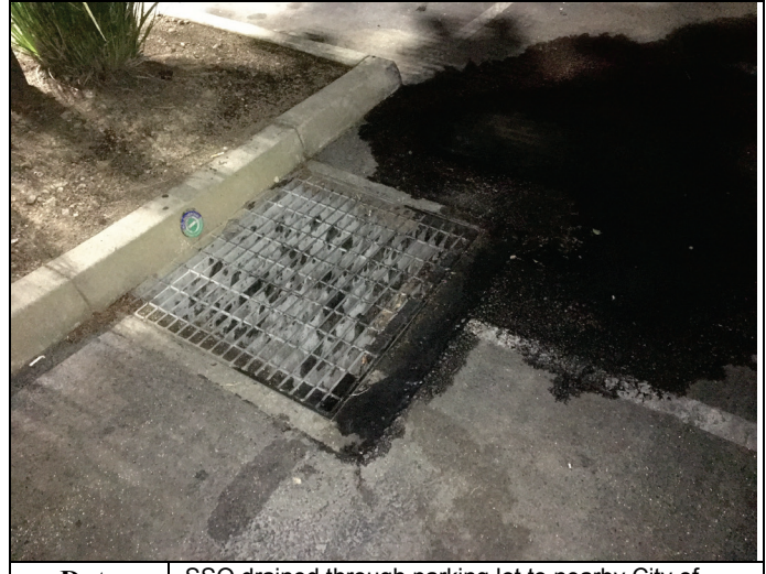
Date SSO drained through parking lot to nearby City of Rocklin storm drain inlet. 5/17/19
