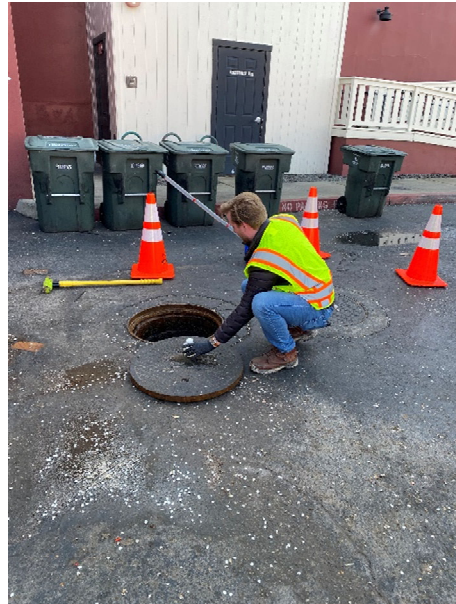
Figure 7 - 03/20/2023 - Grab sample for PH testing.
