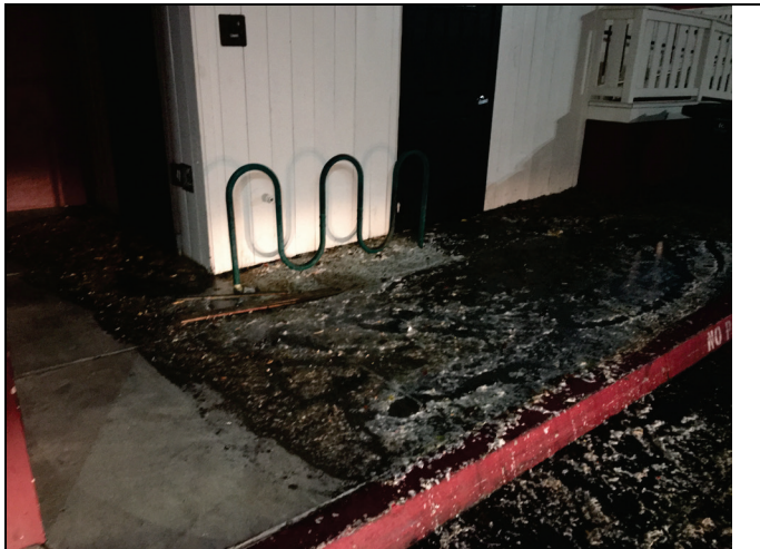
Date SSO containing human waste, toilet paper, fats, oils, and grease. 5/17/19
